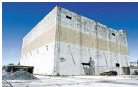
From this nondescript concrete building, the Air Force monitored the activities of enemy airplanes.
