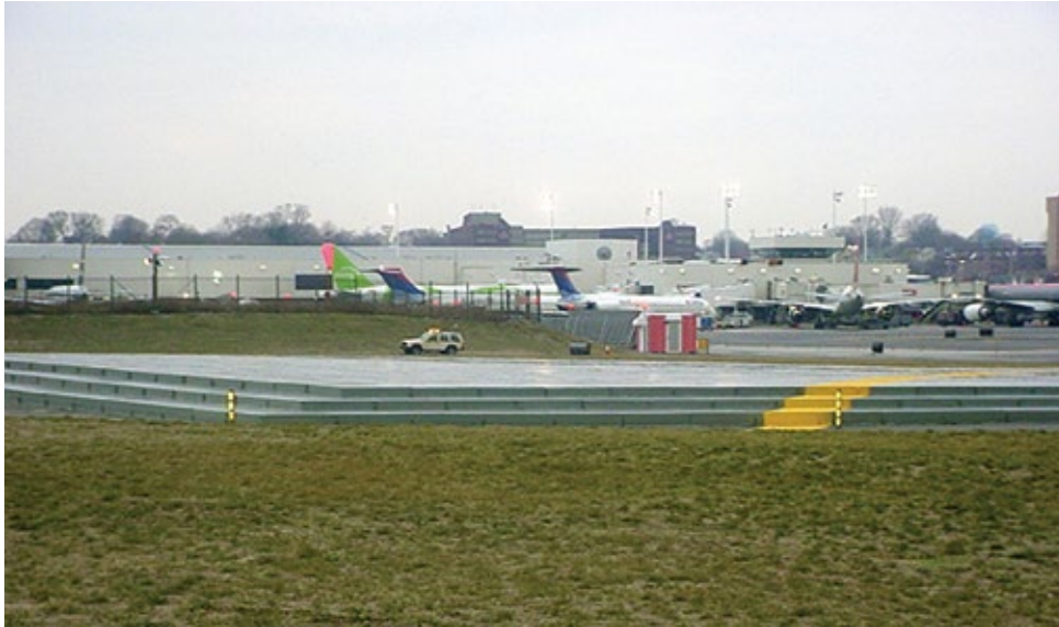
The EMAS (Engineered Materials Arrestor System) bed at the end of LGA's runway 13.
