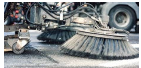
Ramp & Roadway Sweeping
