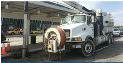
Catch Basin Cleaning & Service
