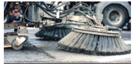
Ramp & Roadway Sweeping
