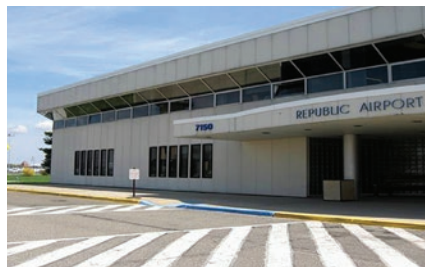
Republic Airport Passenger Terminal
