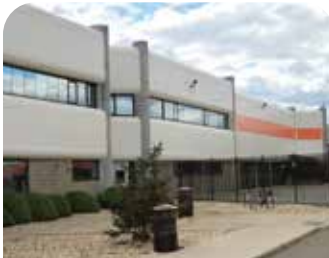
NICE Bus Garden City Exterior Refinishing
