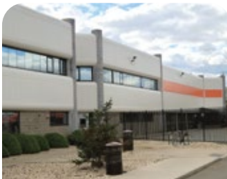
NICE Bus Garden City Exterior Refinishing
