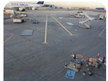
Lead In Striping JFK Airport
