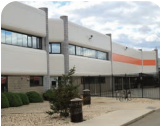
NICE Bus Garden City Exterior Refinishing
