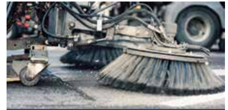
Ramp & Roadway Sweeping
