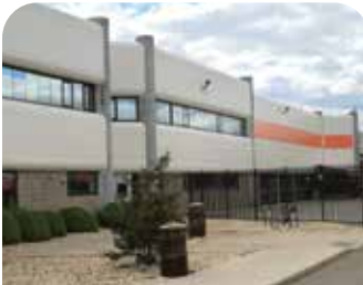
NICE Bus Garden City Exterior Refinishing
