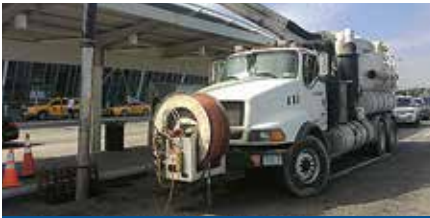
Catch Basin Cleaning & Service
