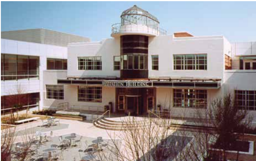
Newark Liberty International Airport, Building 1
