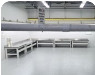
USDA Inspection Area JFKIA
