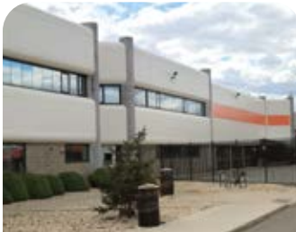
NICE Bus Garden City Exterior Refinishing
