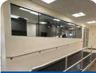
FNBLI Data Center
