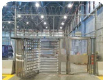
Access Control Systems JFK Airport
