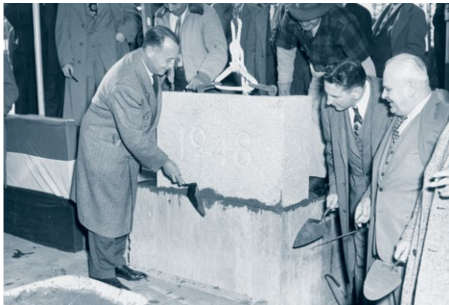
Port Authority Chairman Howard S. Cullman laying cornerstone of Federal Building at Idlewild Airport. D. Rentzel C.A.A. Admin. & Ora Young C.A.A. Regional Admin. looking on. November 8, 1948
