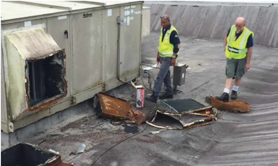
NYNJ Port Authority employees inspecting the condition of a roof at San Juan Airport.
