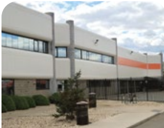
NICE Bus Garden City Exterior Refinishing
