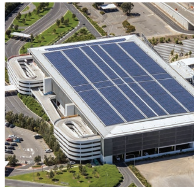
A solar roof array as one shown at Adelaide Airport in Australia is planned for LaGuardia
