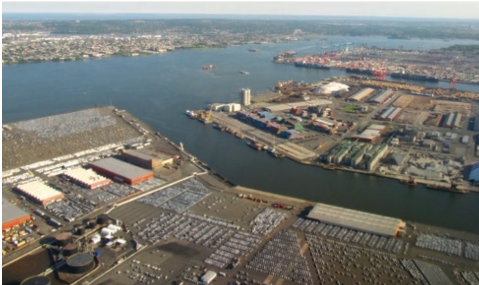
Port Newark–Elizabeth Marine Terminal
