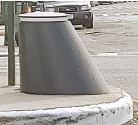
Business owners in the area placed a portable traffic barrier over the DOT-installed "Bollard" that has drivers fuming.
