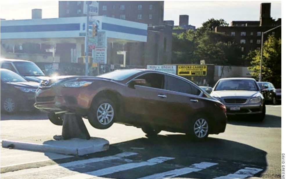
The 2-foot high "Bollard" installed by NYC DOT have been snagging cars, causing damage to vehicles and causing drivers to pay for tow-trucks to remove them.
